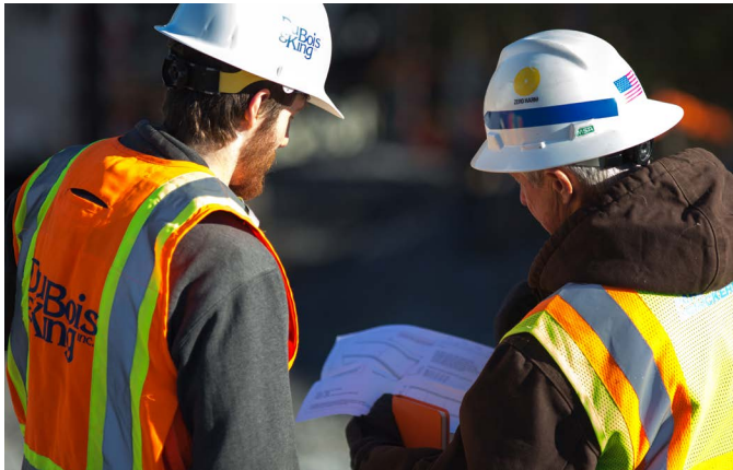
D&K collaborated with WSP's Gordy Eastman on recent rail culvert replacement projects in the Champlain Valley.
